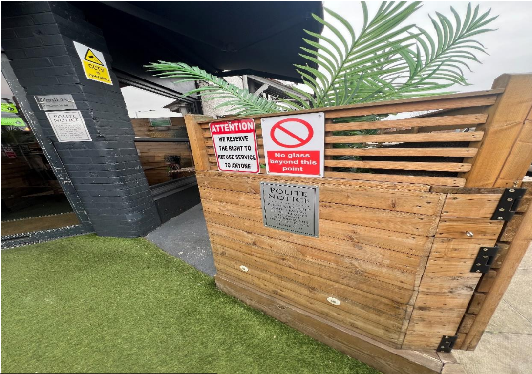
Front Entry Point
